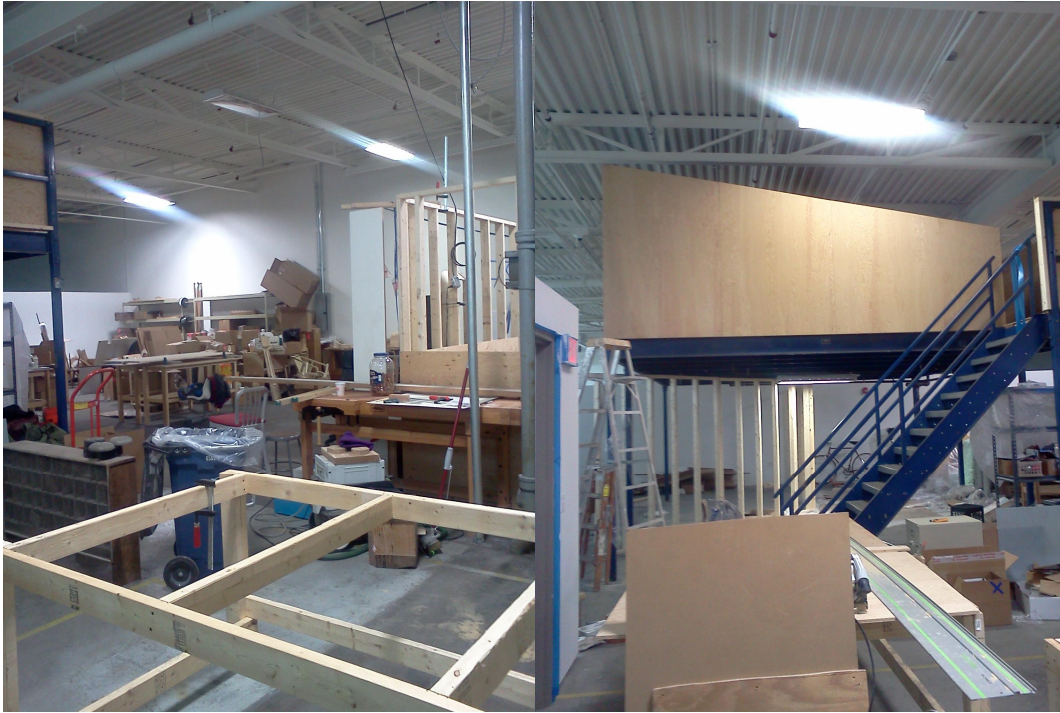
Views of the new Keeseh Studio under construction. Photos: Ned Quist
